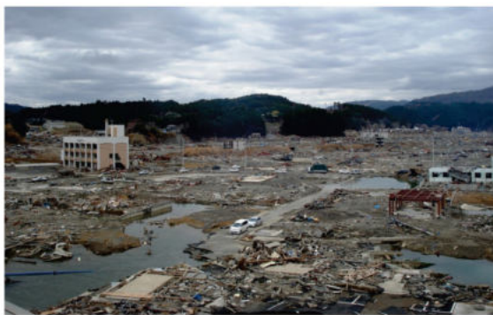
Figure 2-22 Scene of near-total devastation in Minamisanriku, Japan, 2011 Tohoku tsunami (photo courtesy of I. Nistor and ASCE, from Chock, et al., 2013b).
