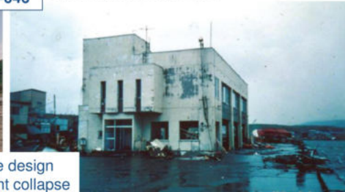
Figure 2-13 Examples of reinforced concrete structures that survived the 1993 Okushiri Tsunami: vista house at Cape Inaho (left); and fish market in Aonae (right) (photo courtesy N. Shuto).
