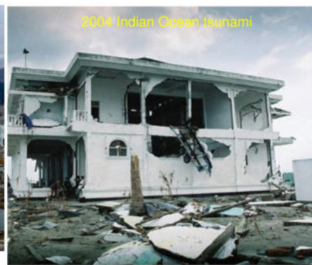
Example of surviving reinforced concrete mosque in Uleele, Banda Aceh (photo courtesy J. Boreiro).
