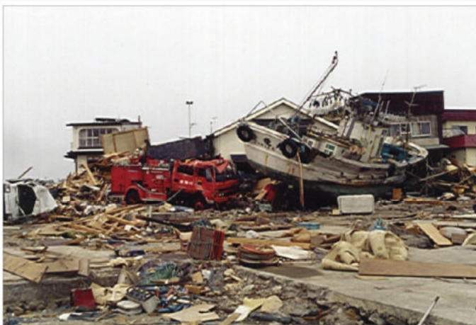
Figure 2-12 Damage caused by impact from water-borne debris (fishing boat) in Aonae, Japan (1993 Okushiri Tsunami) (photo courtesy J. Preuss).
