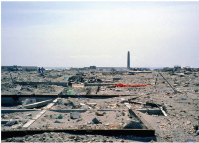
Figure 2-10 Total destruction of a group of wood-frame houses in Aonae Village, Okushiri Island, Japan (1993 Okushiri Tsunami).
