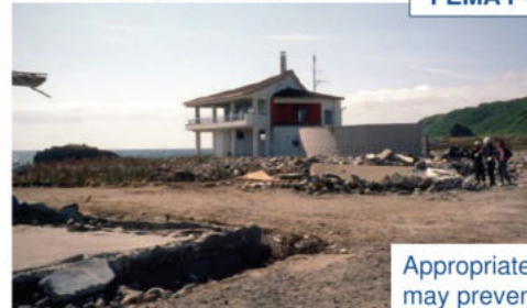
Figure 2-13 Examples of reinforced concrete structures that survived the 1993 Okushiri Tsunami: vista house at Cape Inaho (left); and fish market in Aonae (right) (photo courtesy N. Shuto).
