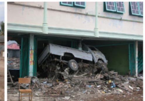
Figure 2-16 Examples of waterborne debris from the 2004 Indian Ocean Tsunami (photos courtesy of M. Saatcioglu, A. Ghojarah and I. Nistor, CAEE, 2005).
